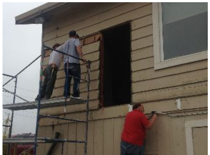
Preparing to close door during workday
