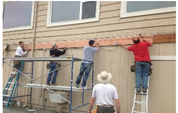
Covering the balcony supports
